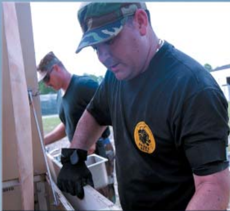
Above: Master Sgt. Kurt Kissel and Tech Sgt. Nathan Hooten hang wash basins on a portable latrine facility they had to assemble during the exercise.
